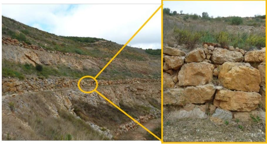
Stone wall construction consists of various rows of stones piled on top of each other along the length of each bench. The walls with greatest vegetation cover seem to be the most used by fauna.
