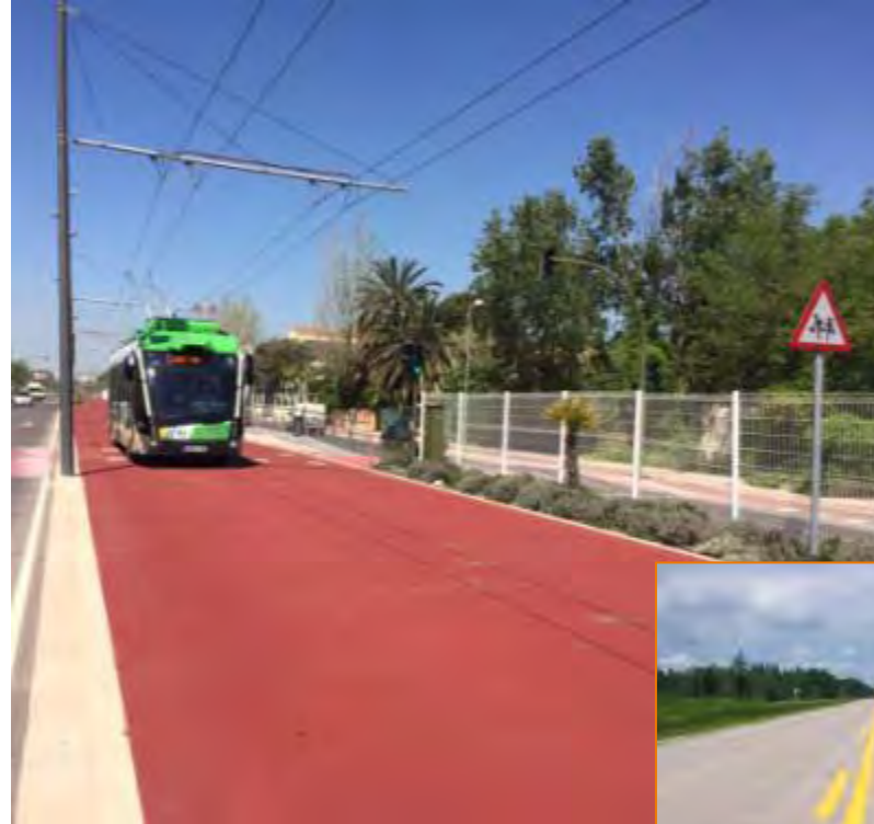
Automated guidance vehicles using a (colored) concrete pavement in Spain
