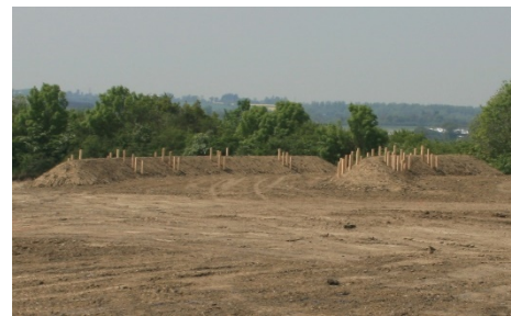
Placing soil to create grassland and mounds
