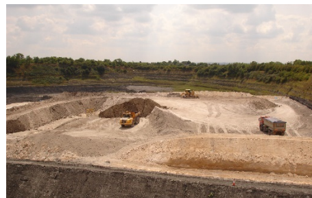
Placing waste in engineered cells
